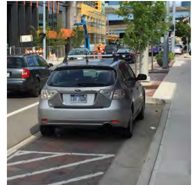
Bridge Street defines on-street parking with colored brick pavers and bulb-outs.
