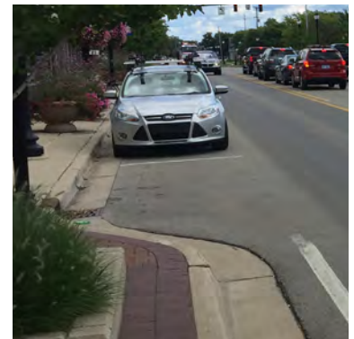
The City of Grandville defines on-street parking with striping and bulb-outs.
