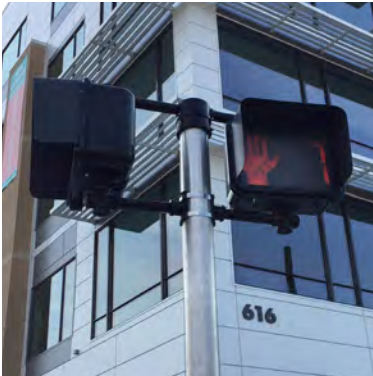
Crossing signals should include a countdown which notifies the pedestrian when the signal will change.
