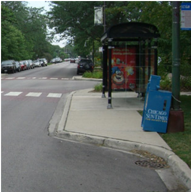
A bus bulb can be incorporated into a bulb out near an intersection.
