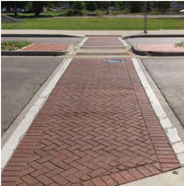
A midblock crosswalk on Division Avenue enhances pedestrian connectivity and provides a safe crossing.
